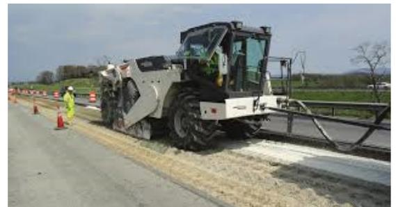
Calciment Is Applied to Stabilize the Underlying Foundation
